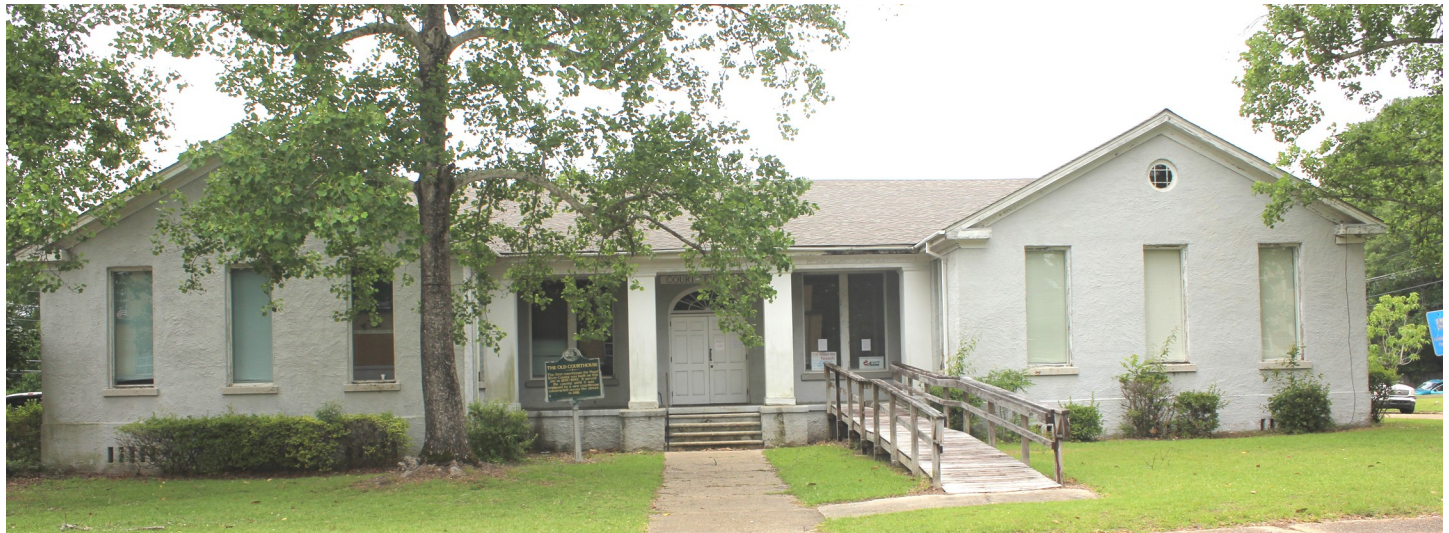
The old Pearl River County Chancery Court Building in Poplarville, with structural and security issues, is expected to be torn down.
